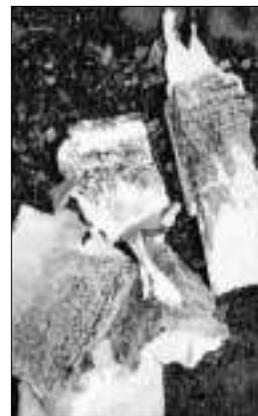
*The extensive moisture and mildew staining in the top photo turned out to be harboring microbial spores, dangerous to my clients.*
