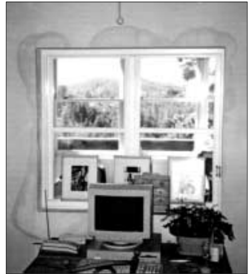
The extensive moisture and mildew staining in the top photo turned out to be harboring microbial spores, dangerous to my clients.
